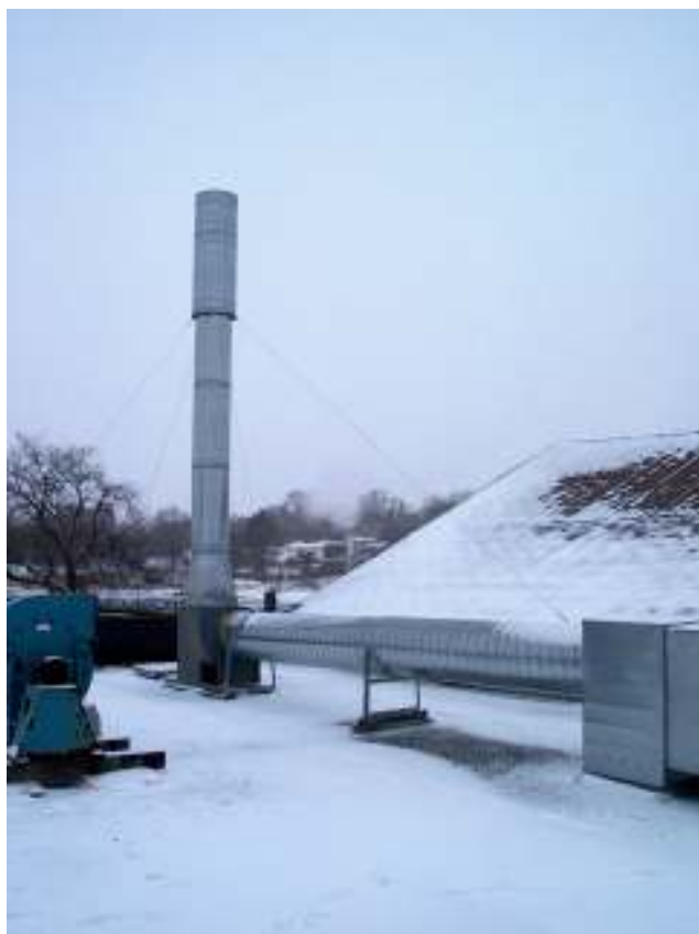
Typical exhaust blower serving fume hood. Take care of it, it is your lifeline.
